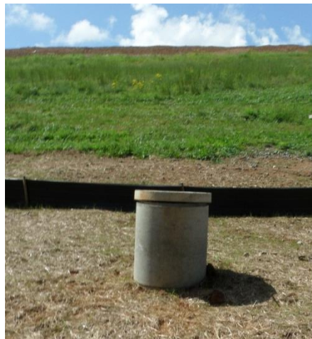
Figure 38. Leachate monitoring well where R. Petty was standing during the earthquake. The soft clay around the well got softer as a result of the earthquake shaking.
