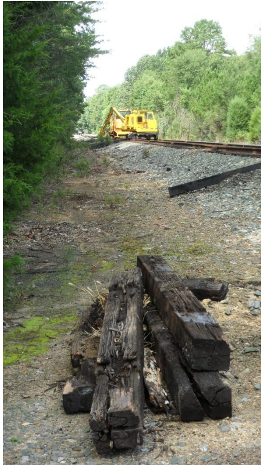
Figure 23. Crew replacing railroad old ties (38.019538, -77.978724).
