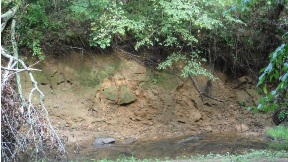
Figure 10. Slump in the bank of the S. Anna River near the Yancy Mill (37.938495, -77.983203).
